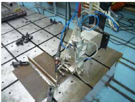
Fig.1 Overview of laser arc hybrid welding for fatigue test specimen
